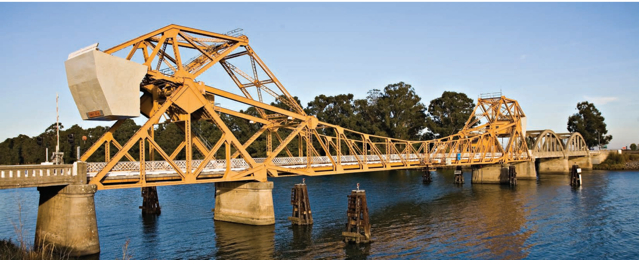
Isleton Bridge / Delta Protection Commission
